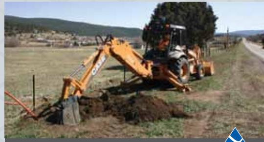
Backhoes are used to dig trenches for new fiber optic lines.
